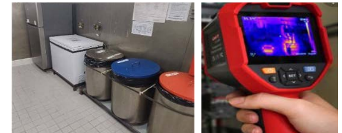
Supply of dedicated freezers for storage of food waste
